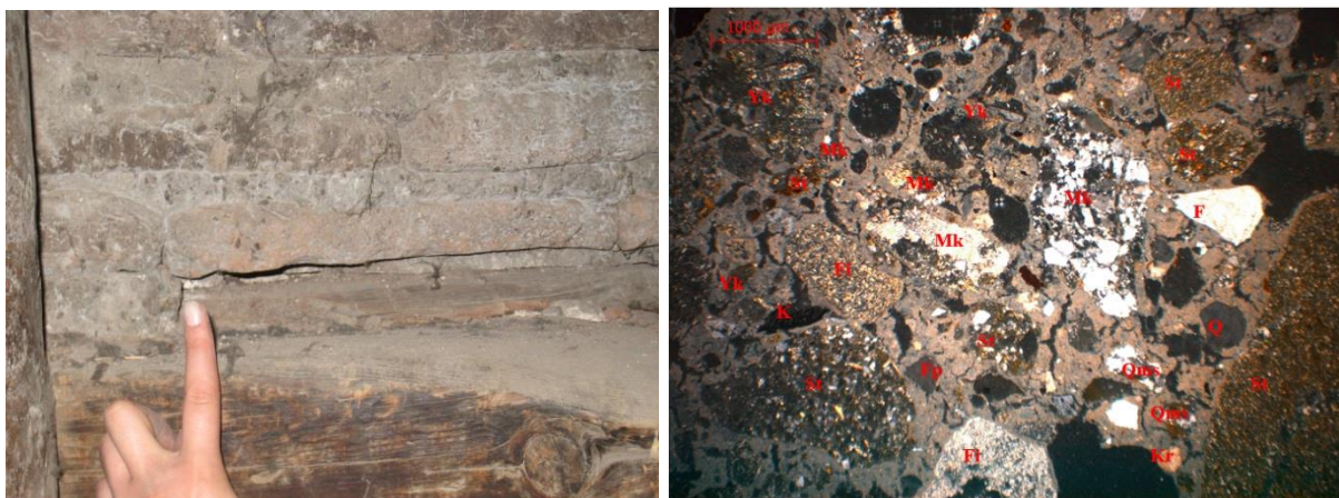
Figure 5. Lime mortar between wood and bricks on the steps of the minaret (left)
