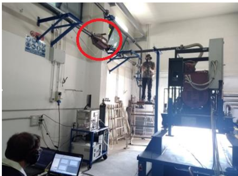
Figure 5. Diesel Genset mockup, DOC converter rounded in red.
