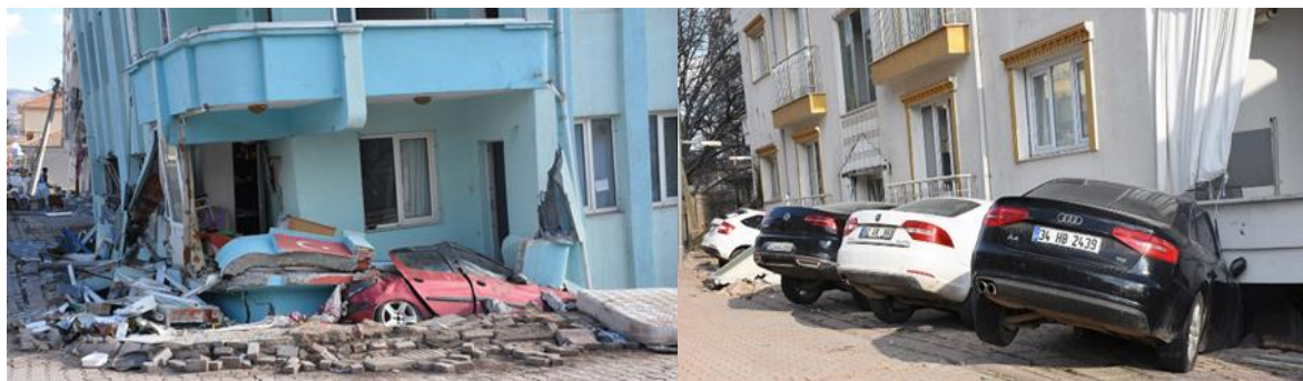
Figure 3 Liquefaction-related building collapse (SSB Post-Earthquake Assessment Report, 2023)
