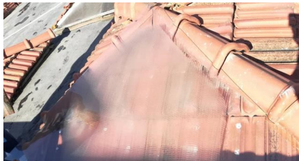
Figure 9. Roof with transparent insulation
