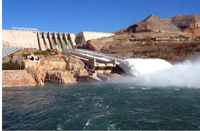
Figure 1. Hydroelectric power plant(WEB2,2018)
