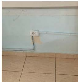
Electricity sockets that can be reached by children
