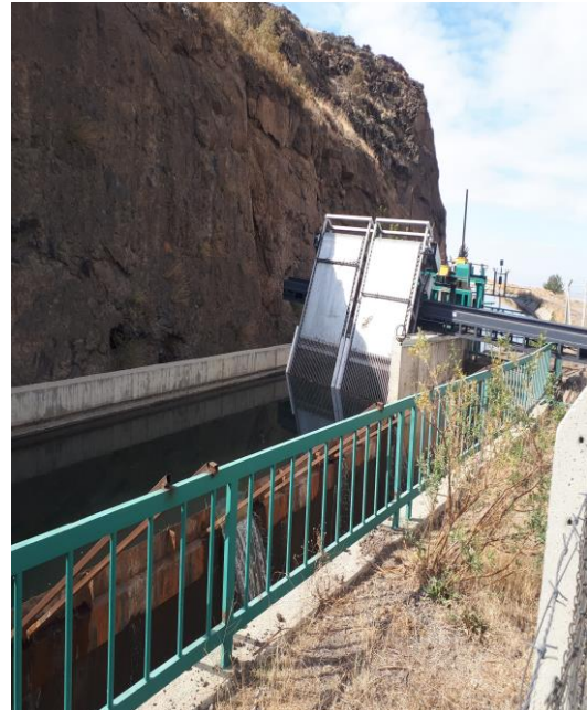
Figure 6b. Mechanical bar screen field application
