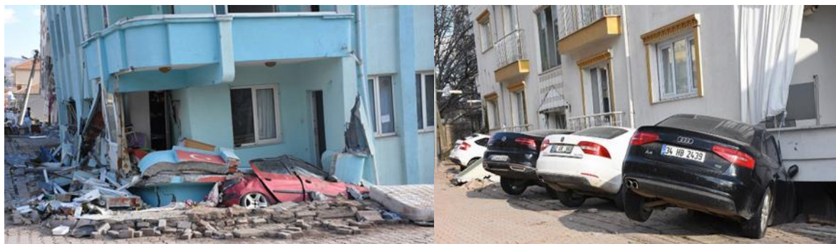
Figure 3 Liquefaction-related building collapse (SSB Post-Earthquake Assessment Report, 2023)
