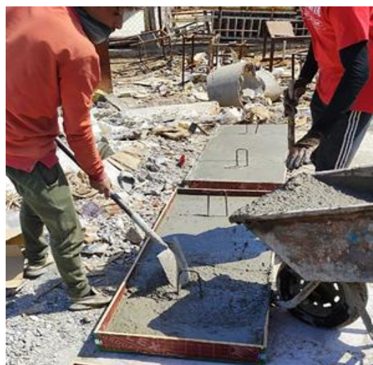
Figure 4. Details of the slab molds
