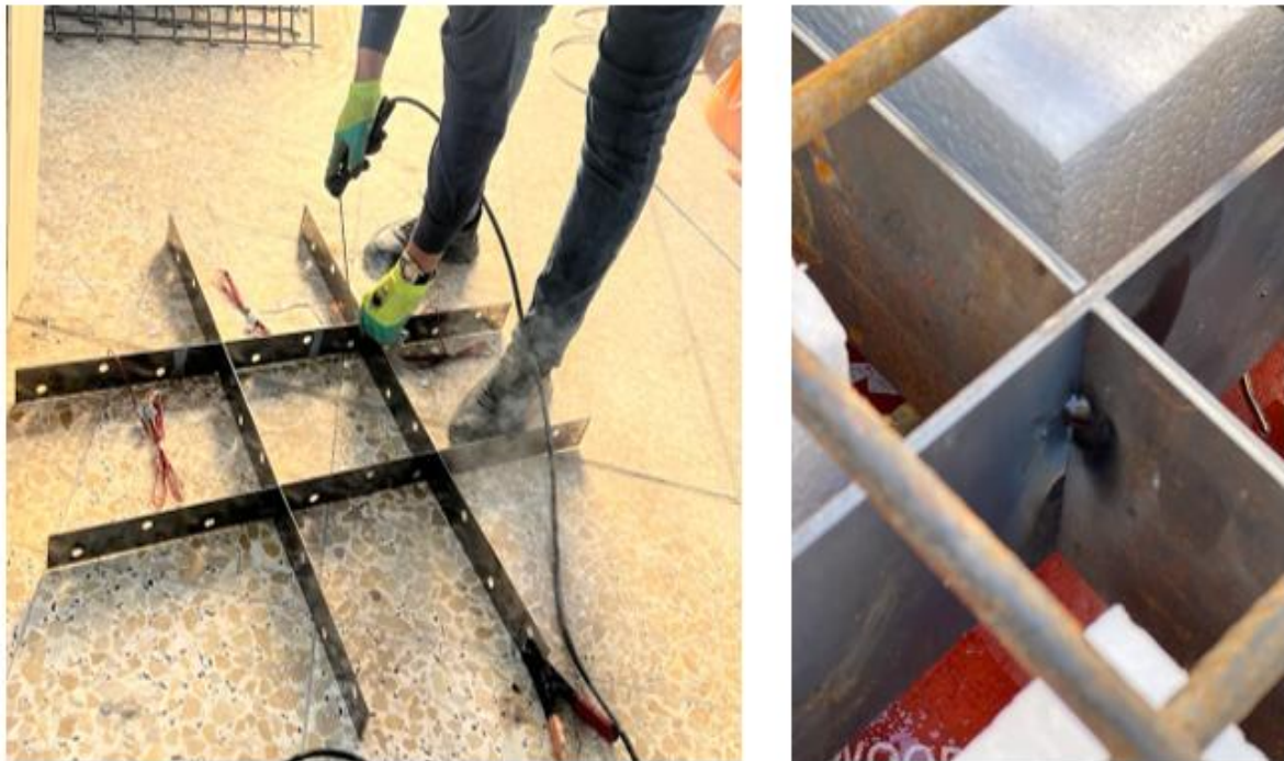
Figure 8. Details of the welding line in steel plates
