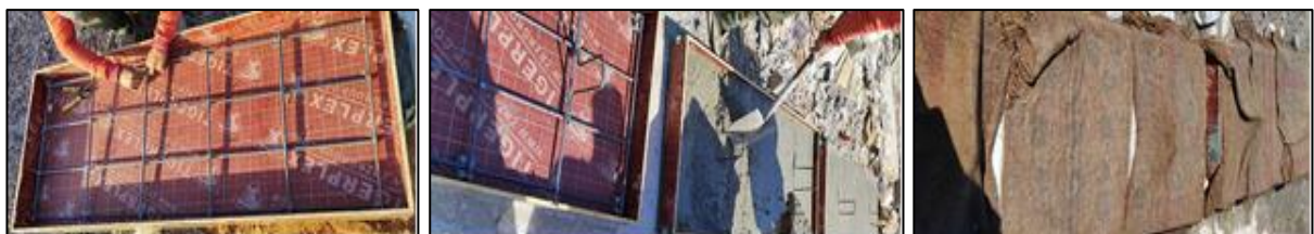
Figure 4. Reinforcement, casting and curing SCC slabs
