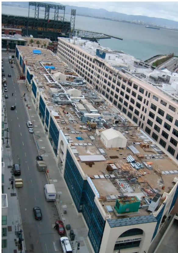
Before the superelevation
